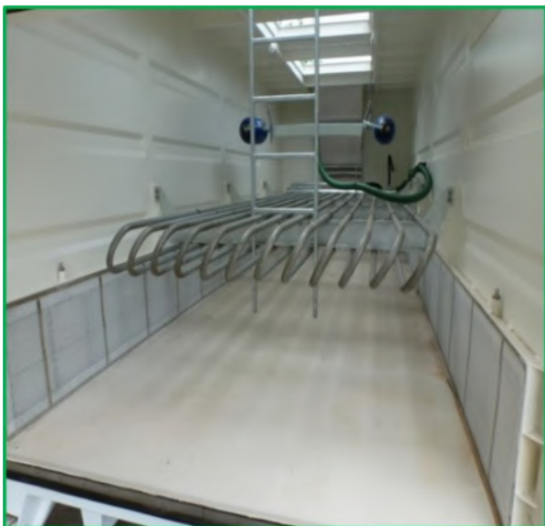
Left: The internal view showing the unique heater coils, access ladder and floating oil skimmer, along the base can be seen the water removal filter screen system.
